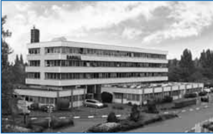
Head office Rosny-sous-bois (France)
